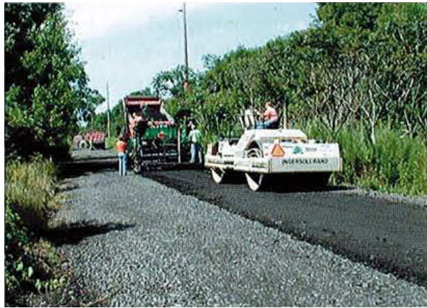
Laying & Compacting the Cinder Trail Base
