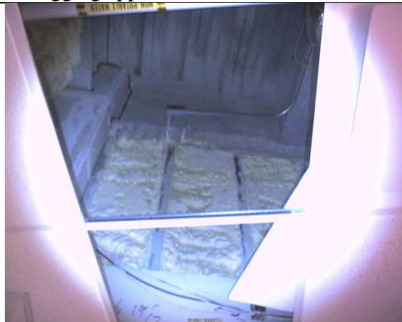
Figure 13 Another location of the showing the air leak at the top of the wall demising wall between garage and conditioned space. The bright vertical lines are infrared reflecting off the shiny steel studs.
