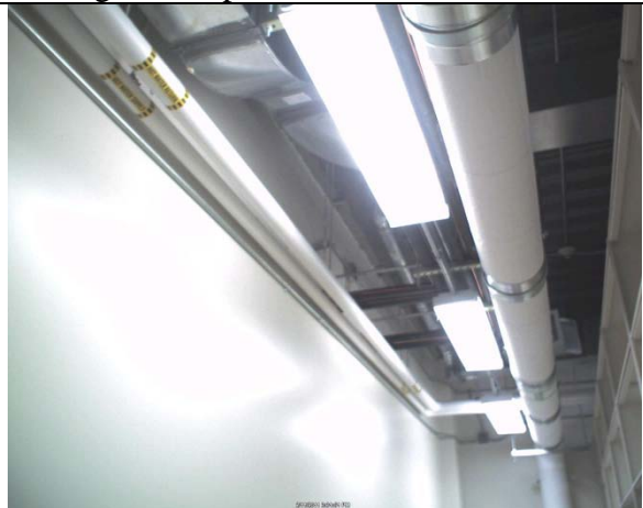
Figure 12 The largest single leak in the building is at the top of the wall separating the garage (with the mesh doors) from the conditioned space. In the IR image the solid portion of the wall shows a uniform,
