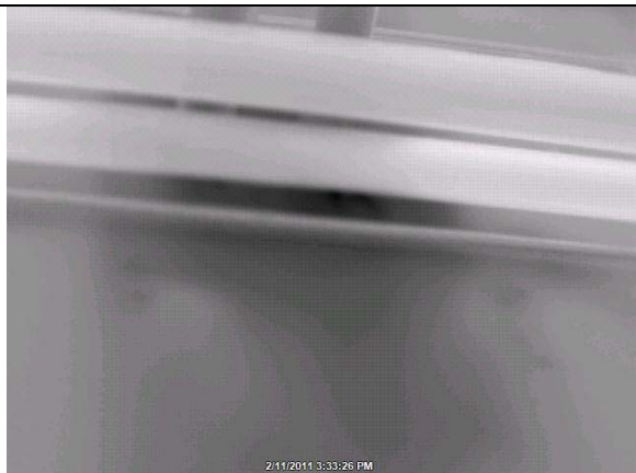
Figure 14 Another location showing air leakage through the fire lagging at the top of the garage demising wall.
