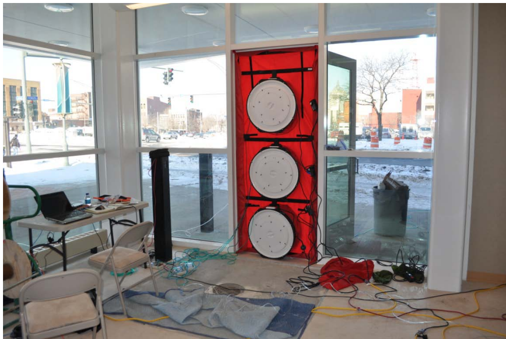
Figure 1. Main lobby fan installation.
