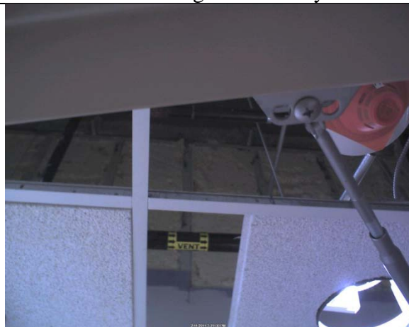
Figure 14 Another location showing air leakage through the fire lagging at the top of the garage demising wall.
