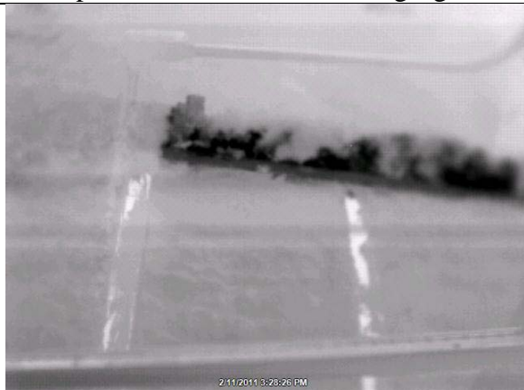
Figure 13 Another location of the showing the air leak at the top of the wall demising wall between garage and conditioned space. The bright vertical lines are infrared reflecting off the shiny steel studs.
