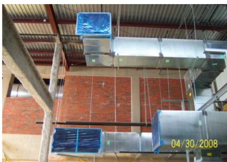
The air handling systems in the building were protected during construction and a building flush-out prior to occupancy was performed to further reduce potential for problems arising during the operational life of the building. The joint efforts of the College, building design team, contractors, subcontractors and suppliers were integral to providing a quality indoor environment.
